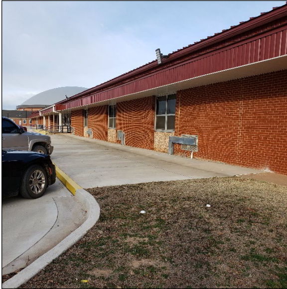
Dome in the background, secure entry vestibule ahead, geothermal system wells at exterior wall
